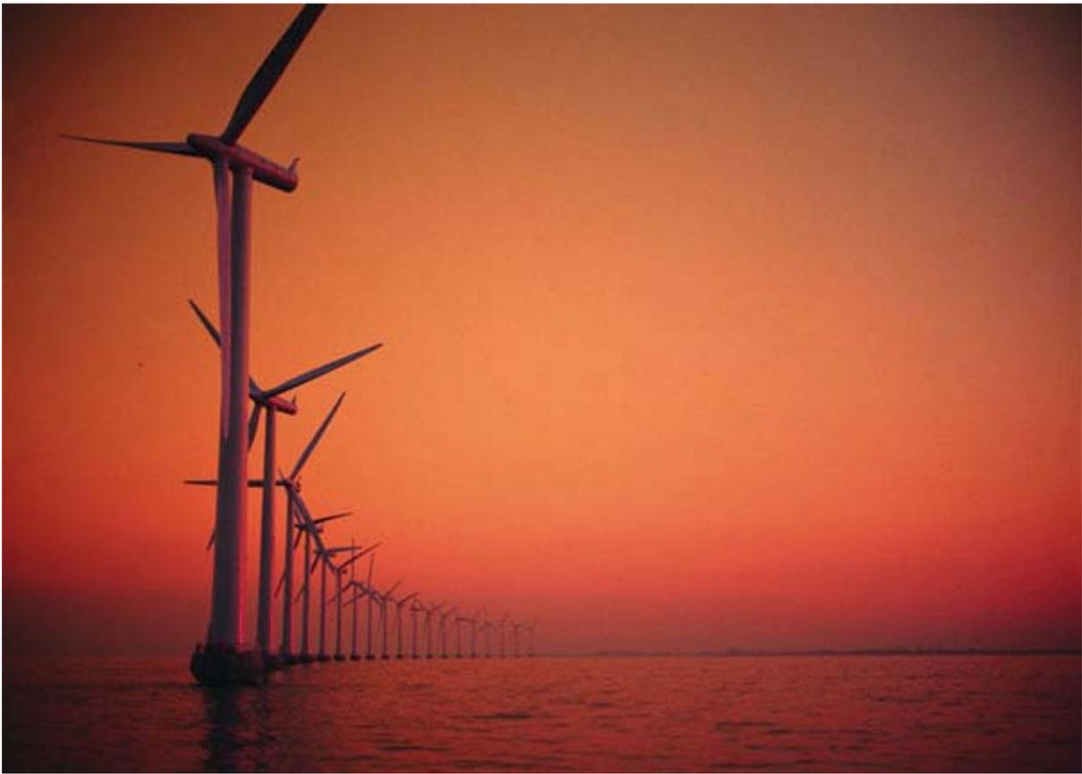
An offshore wind farm at Middelgrunden near Copenhagen, Denmark. Each rotor blade is 36.8 m long.
